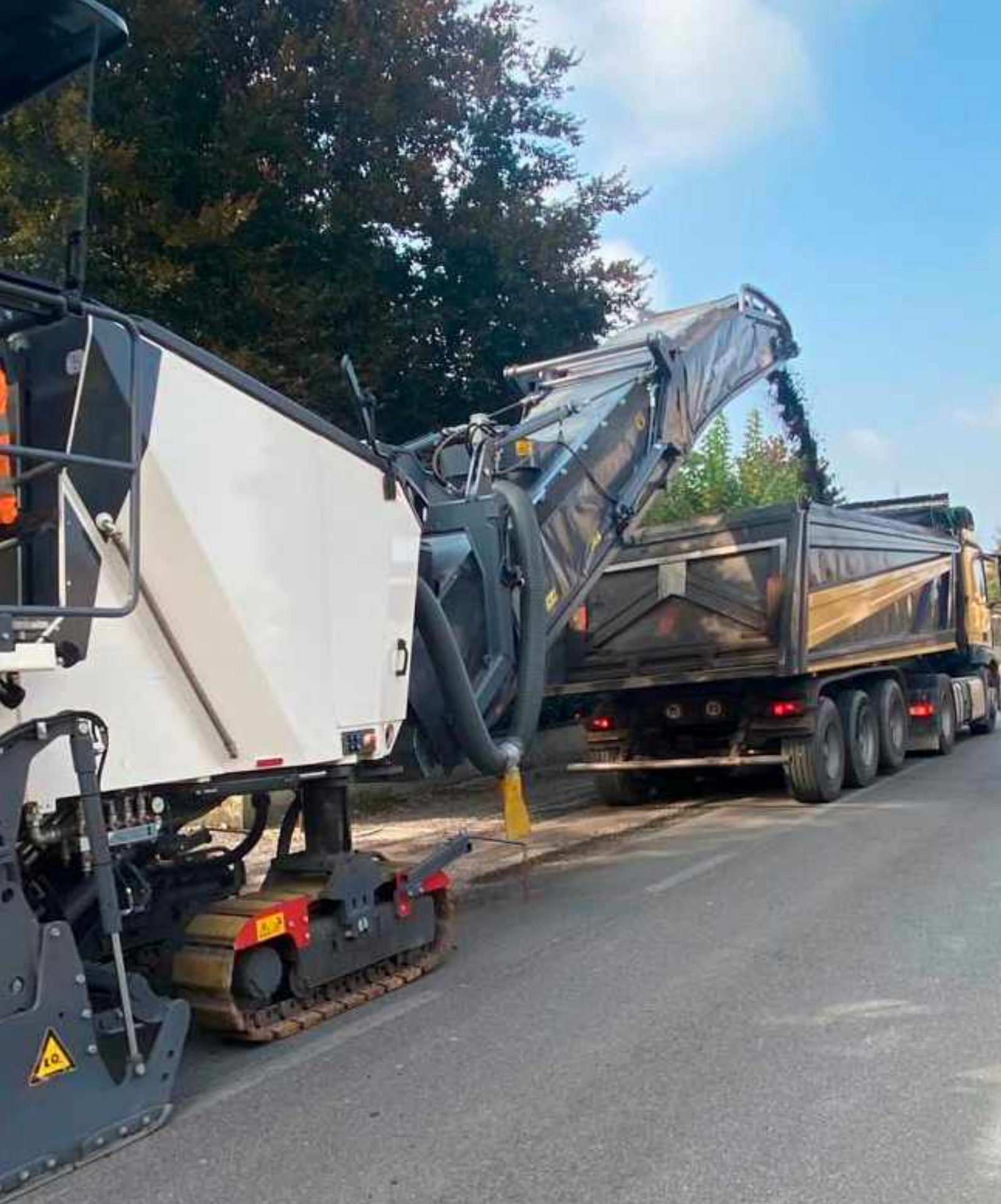
FRESATURA STRADALE road milling
